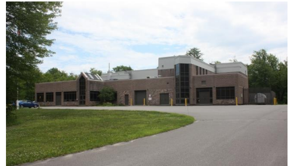
Kirby's Beach WTP
